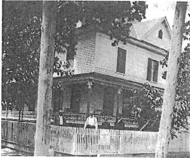
S. B. Whipple Home - Few homes in town were more spacious than this one. It stands today on the northeast corner of Sixth and East Dykes Street. When Mr. Whipple first built the house it had only one story. Later, the second floor was added. This picture was taken in 1909 and shows, left to right, Stephen Whipple, Mr. and Mrs. S. B. Whipple and Dr. R. L. Whipple.
